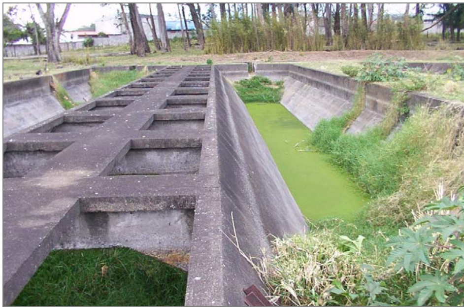
Tanque Imhoff (Biodigestor)
